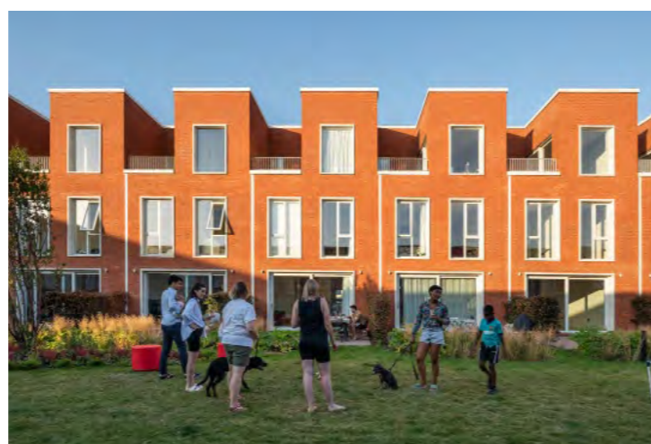
Broken terrace with terraces overlooking an open space.
