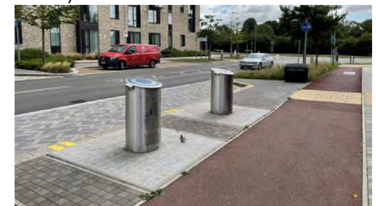
Underground refuse and recycling system, Eddington, Cambridge.
