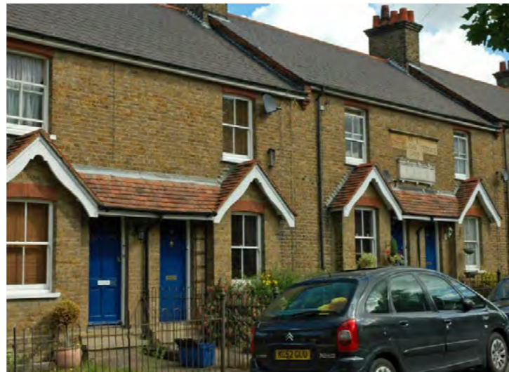
Articulated windows on Oddfellows Terrace, Old Harlow.
