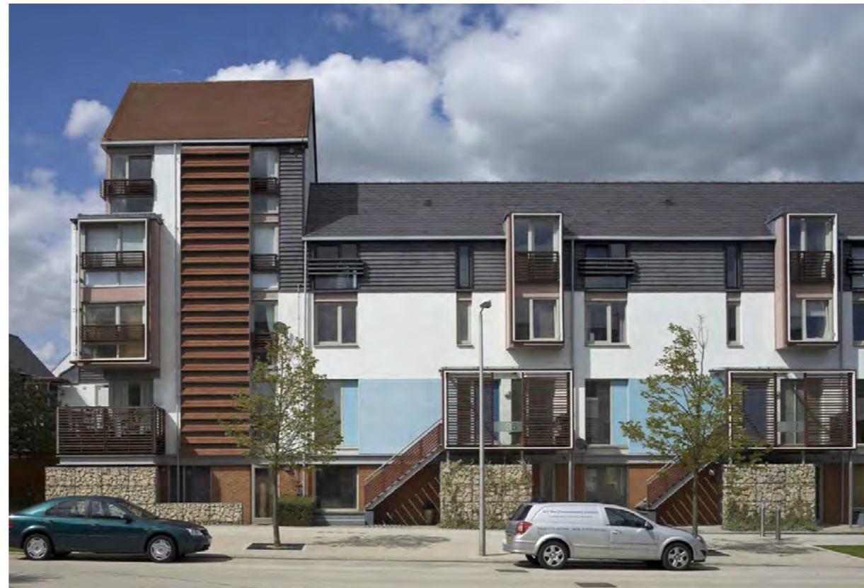
Extra floor to provide height landmark at Abode, Newhall, Harlow by Proctor and Matthews Architects.
