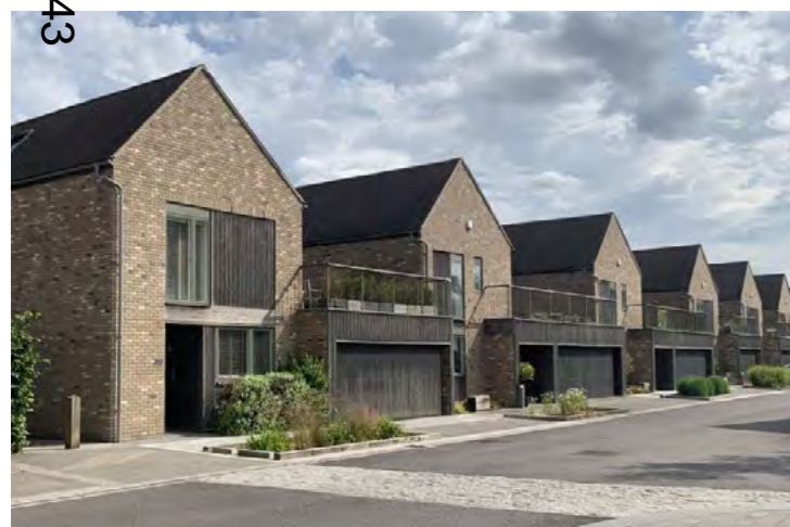
Well integrated enclosed car port with potential for future conversion to living space. Loveden Fields, Hampshire by John Pardey Associates.
