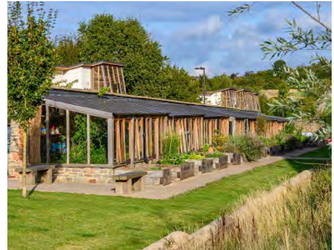
Shared greenhouses and beds at Hanham Hall, Bristol, by HTA Architects.
